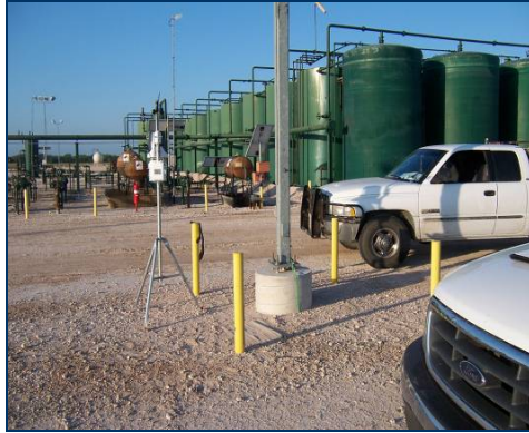
Fig. 10. El Paso Production Condensate Tank Battery (as viewed from the NNE, Kingsville, TX. Note: windsock orientation indicating winds out of the south.
