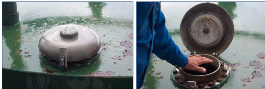
Fig. 11. Thief Hatches closed and opened at Kingsville, TX facility.
